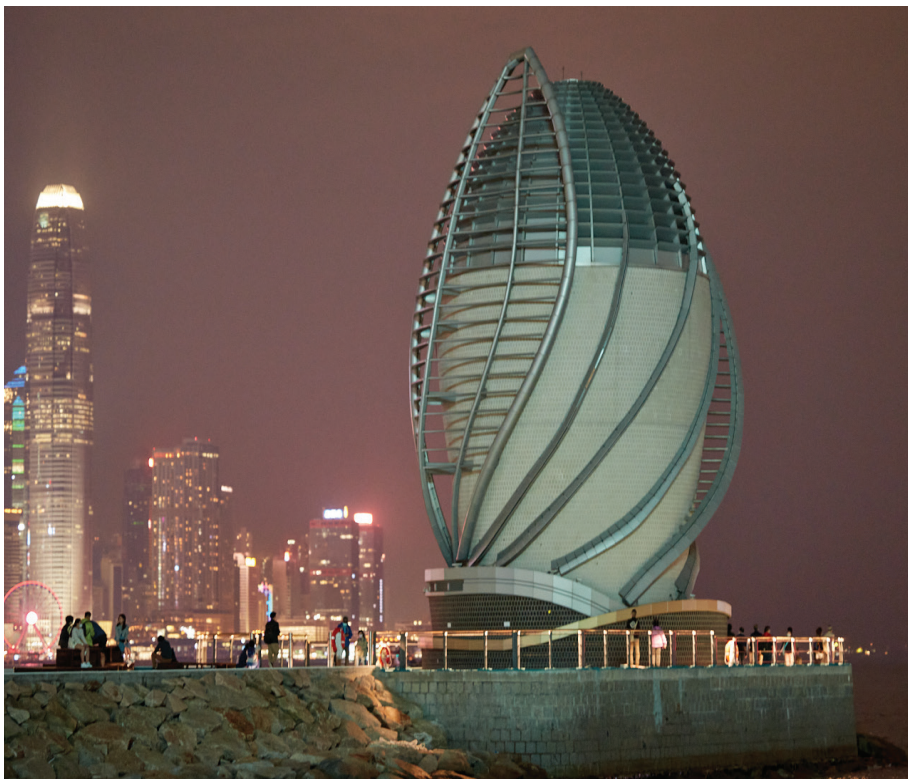
Ventilation Building of Wanchai Bypass Alex W.H. Cheung
