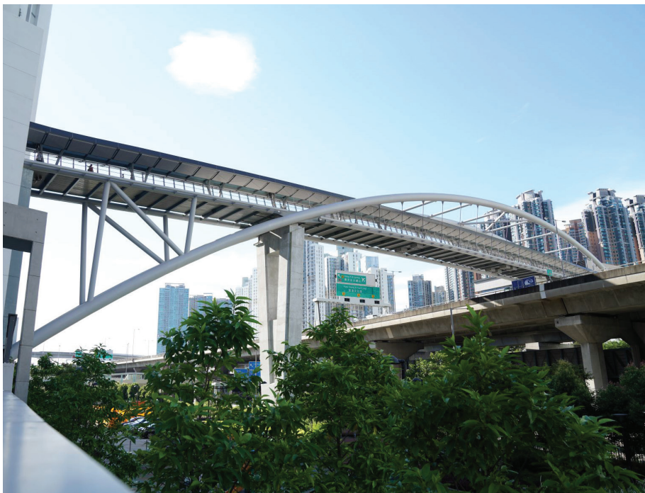
Smart Footbridge with Innovative Technology Yu Man Mak
